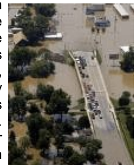
Findlay, Ohio Flood August 2007
